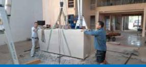
A REID **PORTA**GANTRY lifting and lowering system helped stonemasons working on the altar of a catholic church dismantle the 10-tonne structure safely and easily.
