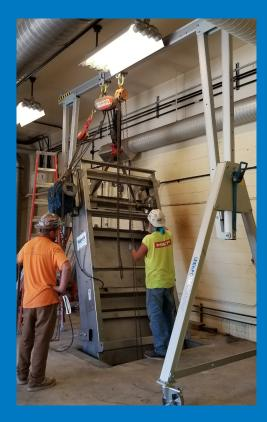
We were able to complete six lifting projects with the Gantry provided from REID, it is great to use onsite, being light and easy to move, assemble and disassemble. REID's **PORTA**GANTRY was the ideal solution for Boller Construction to safely lift, transport and relocate heavy bar screens within restricted access zones in a wastewater facility.
