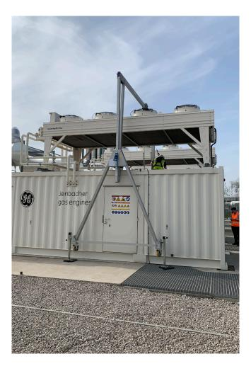
Eurosafe Solutions supplied Conrad Energy with a REID **PORTA**GANTRY which is enabling the Independent Power Producer (IPP) to comply with all the relevant working at height regulations at its Red Scar fast response power project near Preston.
