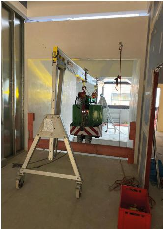
Additionally, each side of the elevator shaft was on different levels with a restricted height, therefore the requirement was for a lifting solution which was suitable for these different levels and can lift up to 3000kg in a restricted space.
